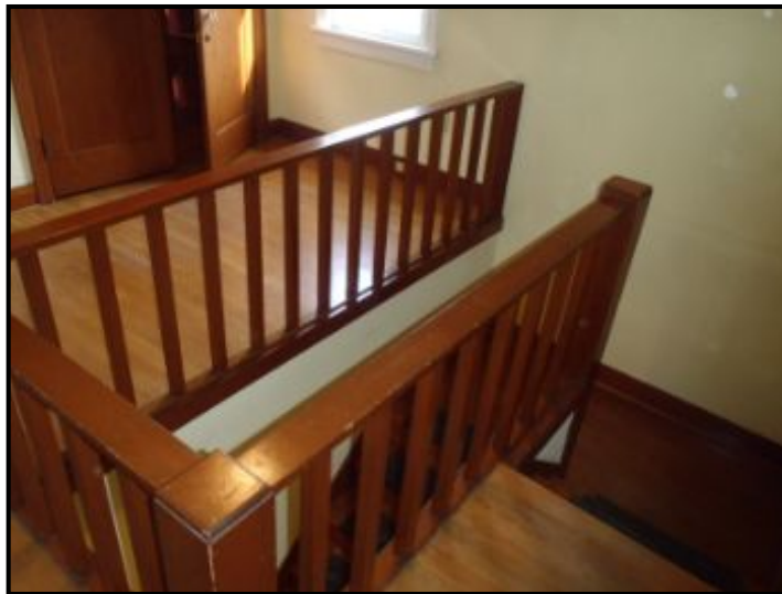
The opening between spindles is over 4 inches wide .
